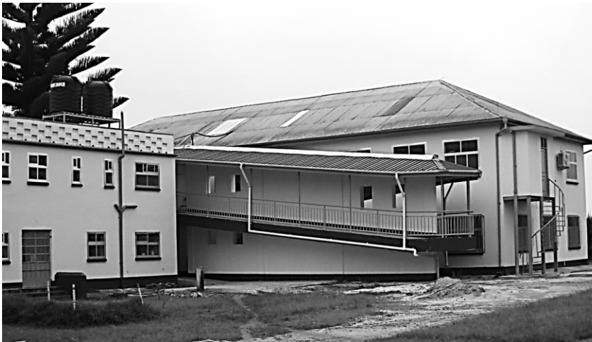
Renovated St. Anna's Health Centre: Picture below: ramp going up to the first floor > Theatre
