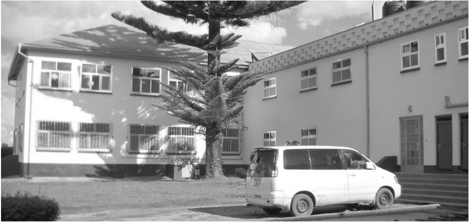
lft. Ground floor = OPD, 1 st floor Maternity / rt. Sanitary Facilities
